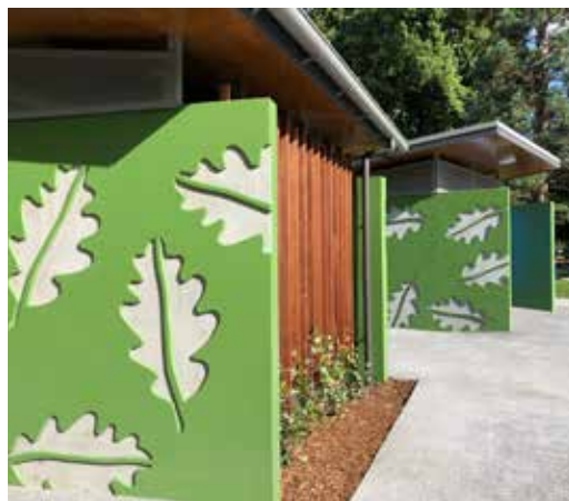
above: Many designers are drawn to using verdant Resene green paint colours on projects that have a direct connection to nature, such as these park toilets, and in combination with other biophilic design strategies. Precast concrete walls painted in Resene Uracryl tinted to Resene Dell, timber cladding and soffits stained in Resene Ironbark and topcoated in Resene Uracryl Clear and steel in Resene Uracryl tinted to Resene Sandstone Grey. Design and image by Citrus Studio Architecture, www.citrusstudio.co.nz. Build by Tims Construction, www.timsconstruction.co.nz. Painting by Steve Olsen Decorator.
