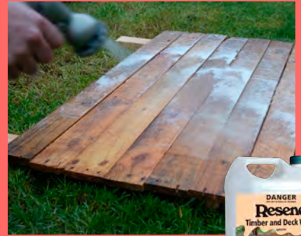
Above: To get started, place your first pallet down on a flat surface and saw off each side stringer. Clean thoroughly with Resene Timber & Deck Wash, using a scrubbing brush to remove any dirt and stains.
