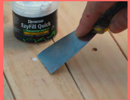
Above: Once your bar is assembled, fill any holes with Resene Ezyfill Quick, then sand and wipe off sanding dust and apply a coat of Resene Quick Dry primer for an even, undercoated surface before painting.
