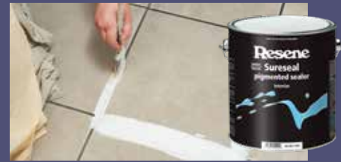
2: Apply one coat of Resene Waterborne Sureseal to the tiles and grout and leave it to dry. Use a cutting in brush for the edges and grout, then a roller for the tiles.
