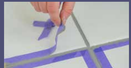
4: Carefully mask around the grout and paint on Resene Walk-on in your grout colour.
