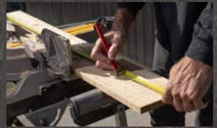
1: Measure and cut the timber components and sand edges. Wipe off sanding dust.
